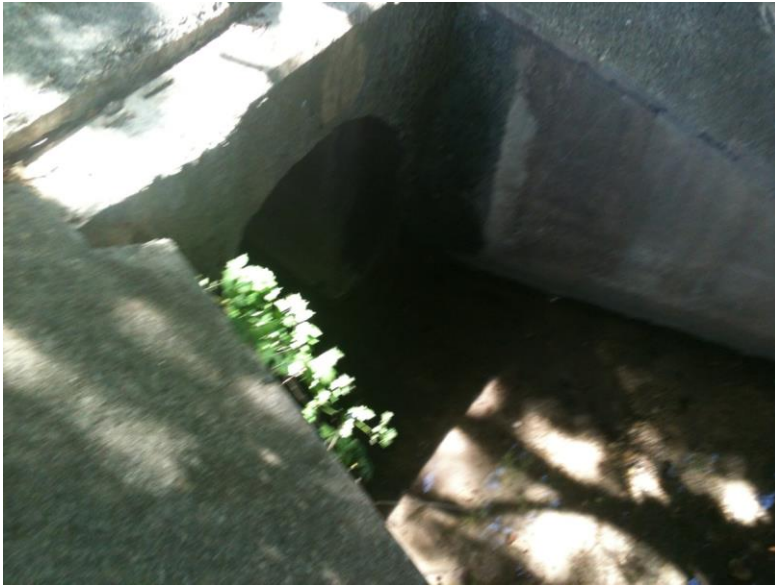
Figure 8-20 Photo of Existing Trail, Culvert, and Proximity to Bridge and River
