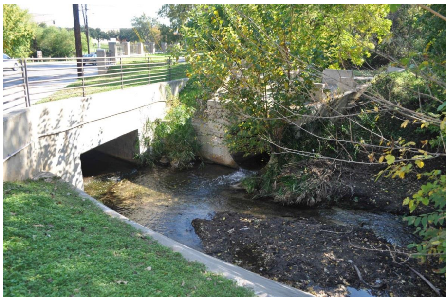
Figure 9-7 Sessom Creek and the Wet Pond Outlet Structure
