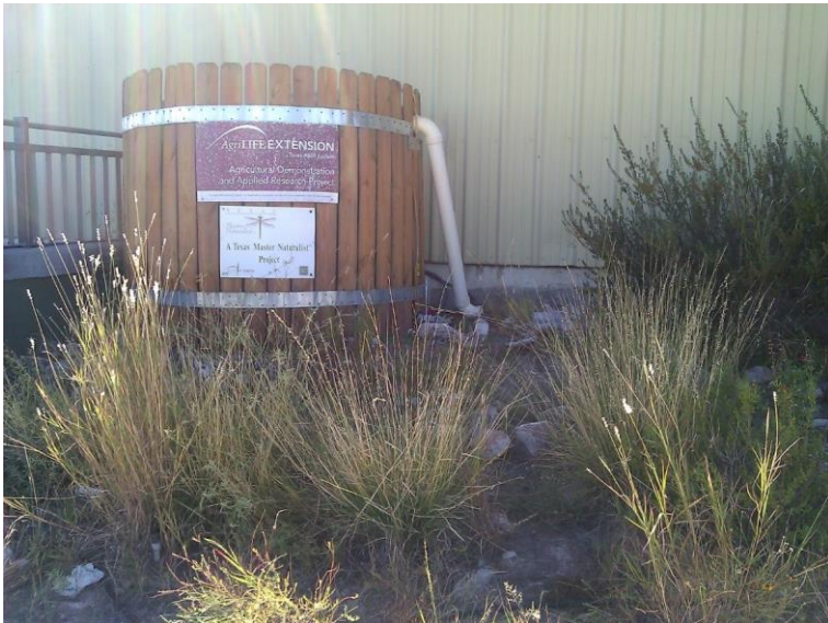
Figure 11-4 Rainwater Harvesting System used to Irrigate Xeriscape
