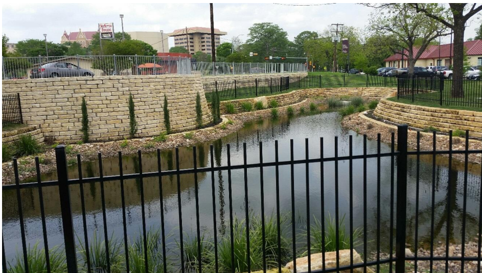
Figure 8-31 Photo of Recently Completed Downtown Water Quality Pond
