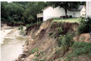
Figure 6-7 Creek Erosion Threatening Home
