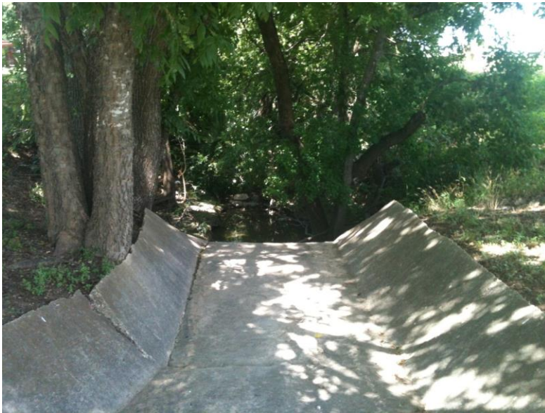
Figure 8-19 Photo of Existing Storm Sewer Outfall Looking Upstream
