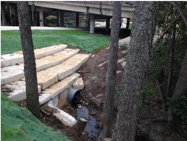
Figure 8-21 Photo of San Marcos Plaza Contributing Drainage and Park Amenities
