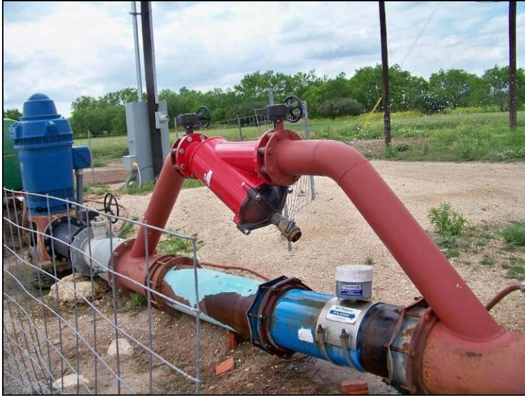
Figure 5. In-line filter sampler.
