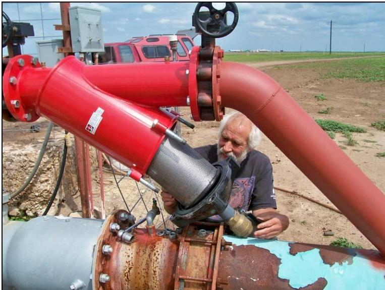
Figure 95. Sampling occurred at Woodley Farms Well No. 2 by examining a removable filter that the landowner had installed in the irrigation line for that purpose.
