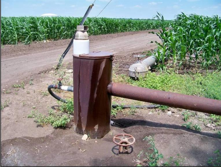
Figure 64. The top of this riser structure was modified with a lid that flips open, allowing access to a net attached to the pipe outlet.
