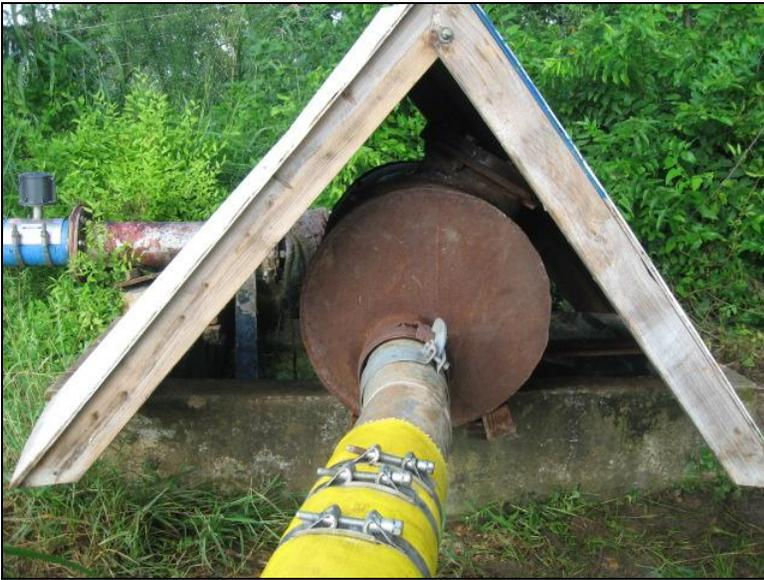
Figure 20. Wooden shade tent over in-line sampler at Aldridge 209 pump site.
