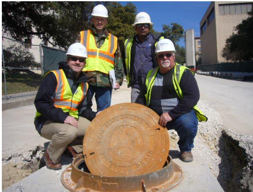
Employees of FPDC and Flynn Construction pose with the first new manhole cover installed on campus.
