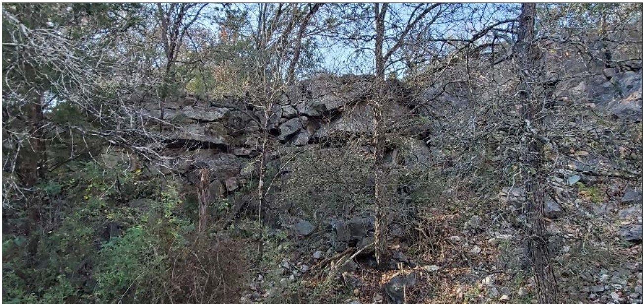
Figure 12. Fractured Marble Falls Limestone (Cmf) upstream of Krause Springs Park
