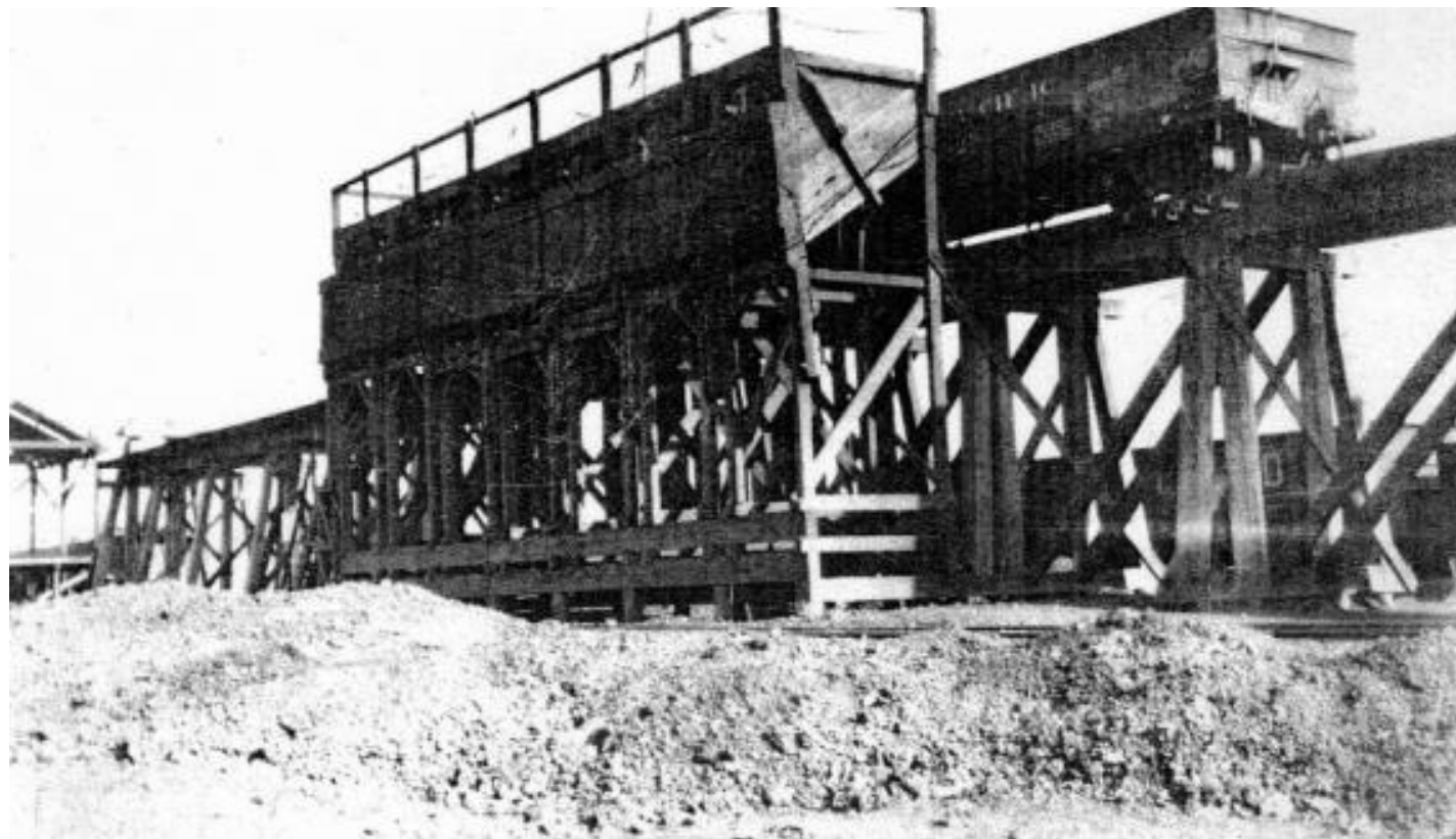
Coal Chute at Toyah, Texas rail yard, ICC files in the National Archives from material that the T&P submitted in 1917
