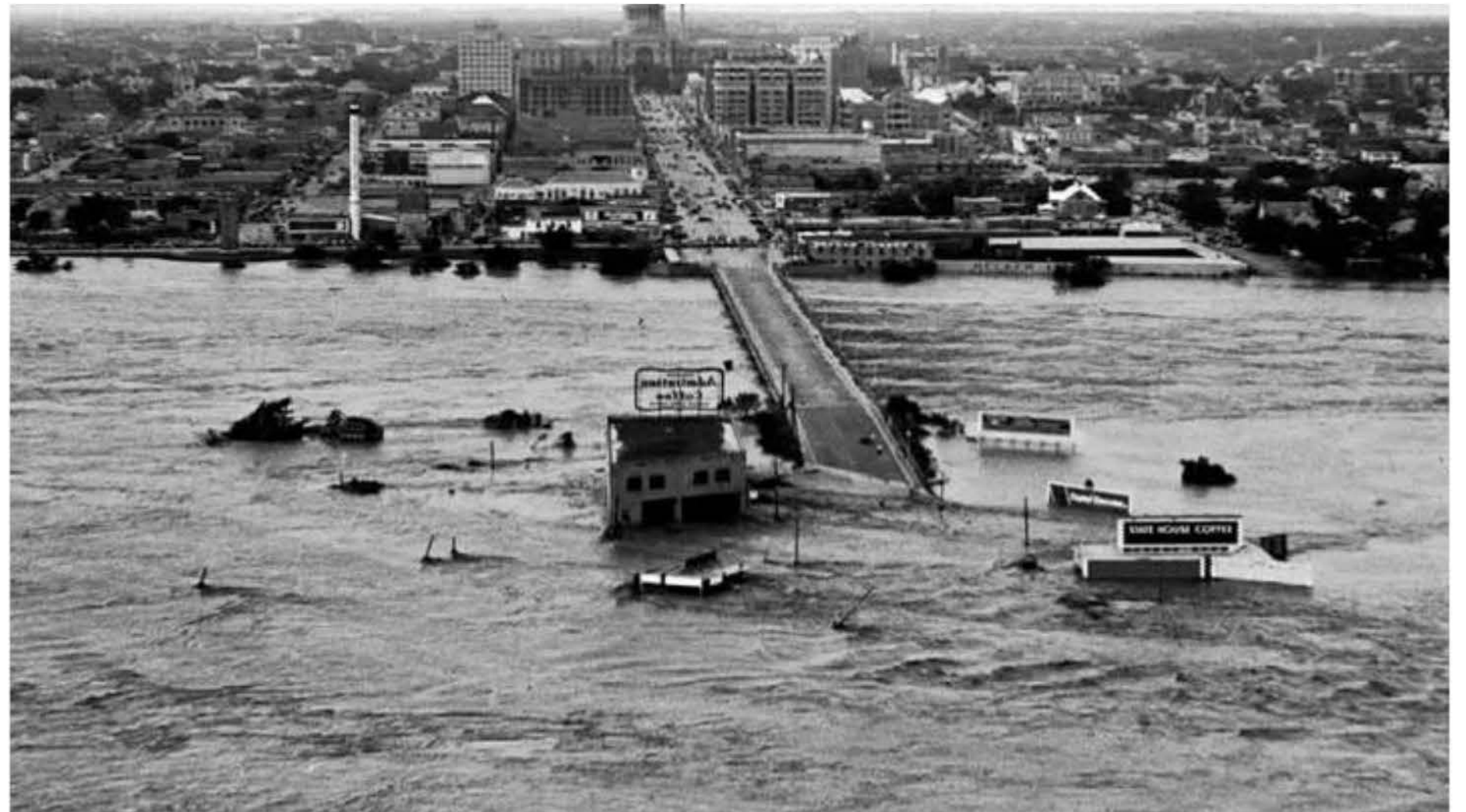
1935 flood photo of Congress Ave in Austin inundated by the Colorado River. Floods in 1936 and 1938 also inundated Congress Ave. Buchanan dam was built shortly after the 1938 flood.
